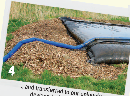
Silt containers can sit up to 2,000 ft. away from ponds, retaining sediments and muck...
